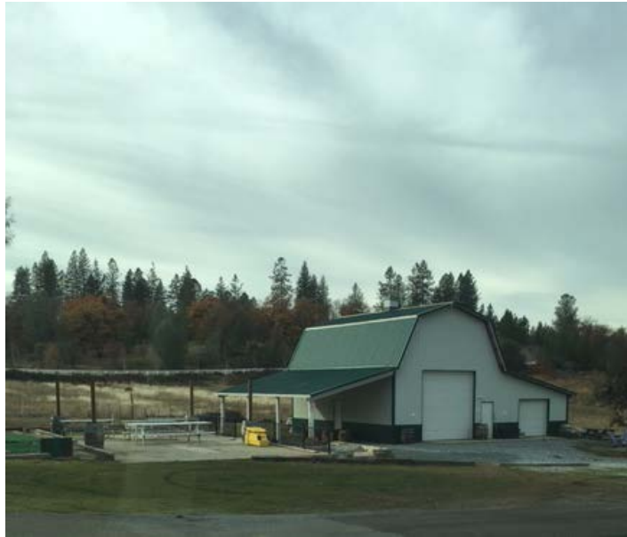
Examples of formal construction with paved parking at Apple Hill.
